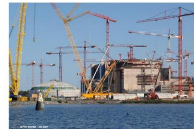
Olkiluoto 3 Preparatory work for the placement of the reactor dome
